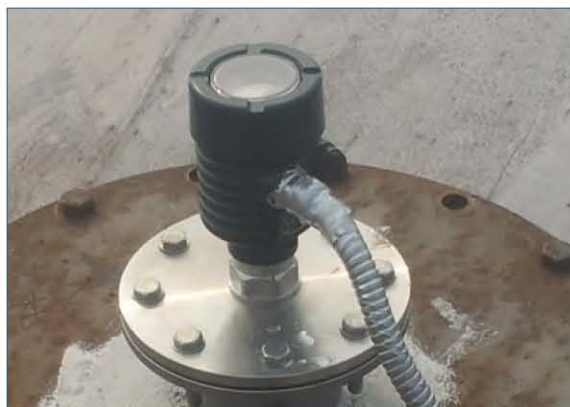
Radar level transmitter in China
